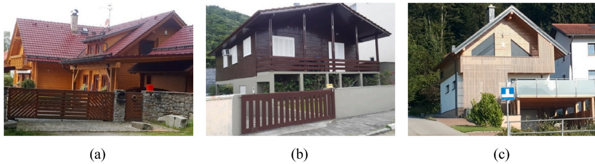
Fig. 1. Versatility in building systems and manufactured materials: (a) solid blocks in a log-home in Czechia, (b) machined wood in a nailed clapboard house in Brazil, and (c) panels in a light-woodframe house in Austria. Photo credits: Victor De Araujo.
