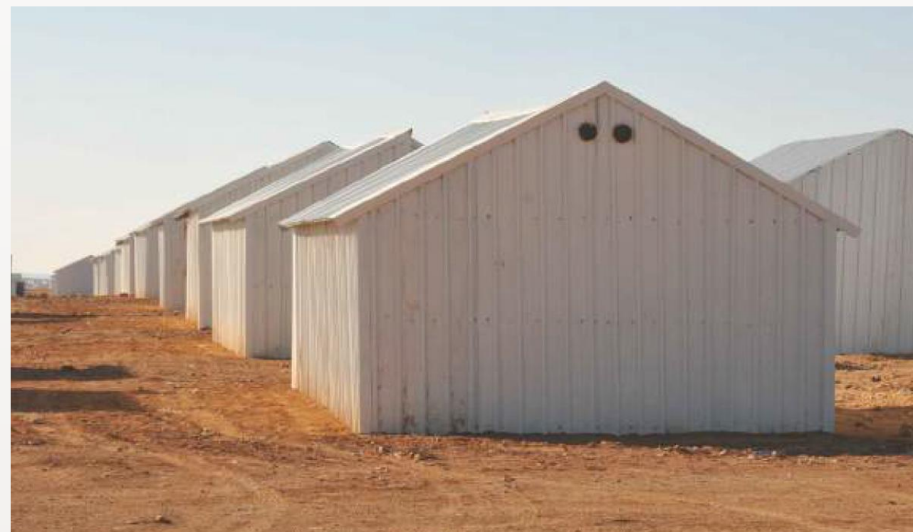
Transitional shelter: 2-4 years durability; steel structure and sheet metal, aluminum foam insulation
