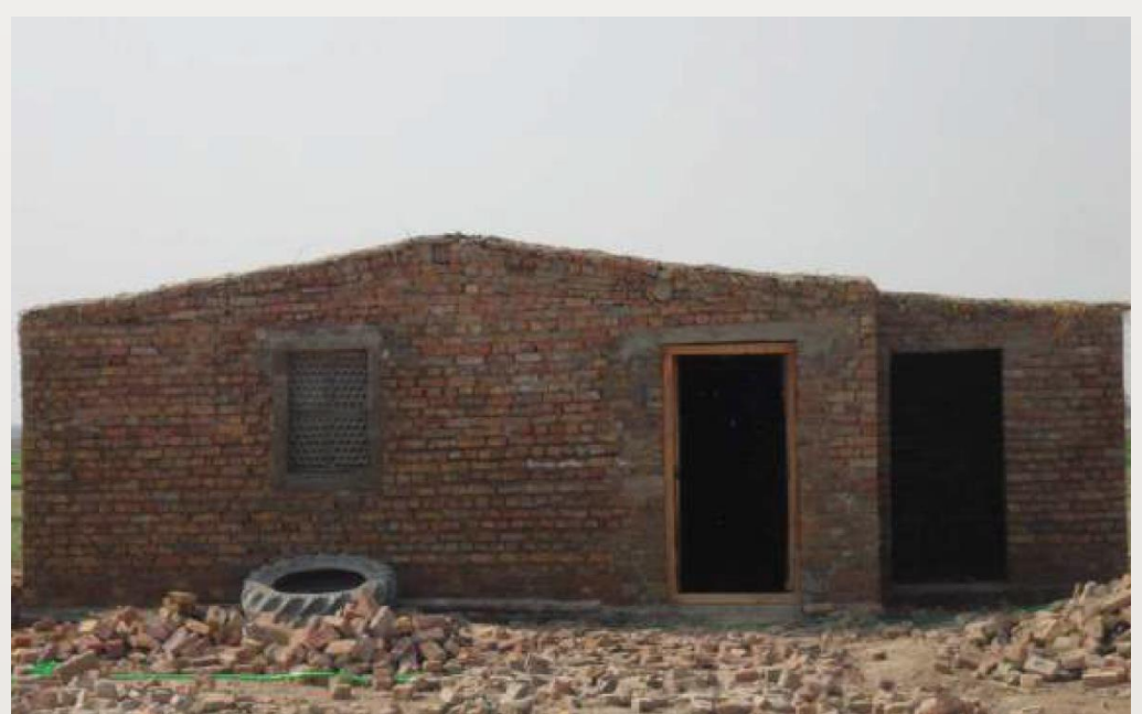
Durable shelter: 10 years durability; brick or concrete tiles, concrete, cement mortar, ceramic tiles or sheet metal (roof), steel beams
