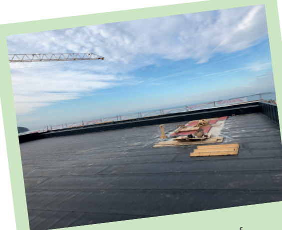
Steam barriers on the main roof Parna zapora na glavni strehi
