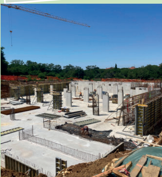
3 Concrete floor slabs in the basement and columns
