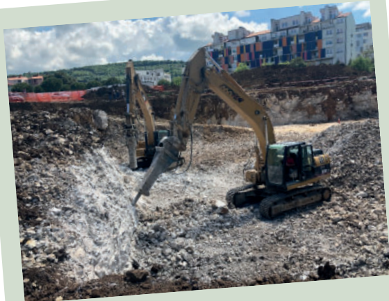
1 Construction pit excavation Izkop gradbene jame
