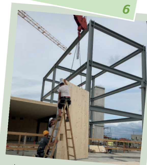
8 Installation of wooden walls and panels (2) Montaža lesenih sten in plošč (2)
