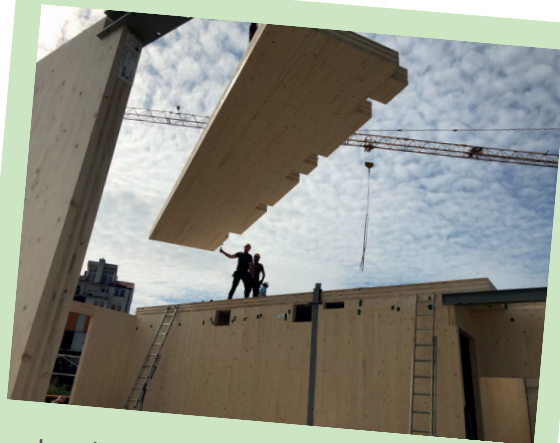
Installation of wooden walls and panels (4) Montaža lesenih sten in plošč (4)
