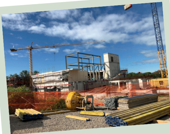
Installation of wooden walls and panels (3) Montaža lesenih sten in plošč (3)
