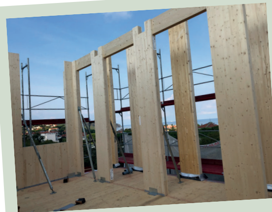
Completion of the building's wooden assembly (1) Zaključek montaže lesenega dela objekta (1)
