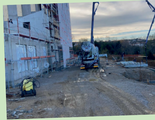
Start of construction for the second building Začetek gradnje drugega objekta
