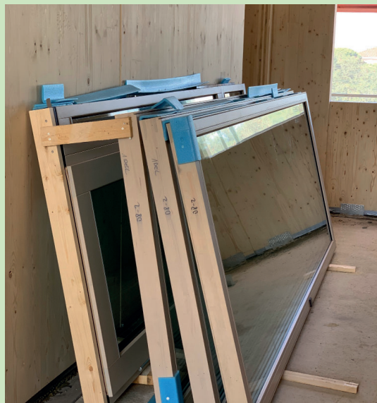
Installation of windows (1) Montaža oken (1)
