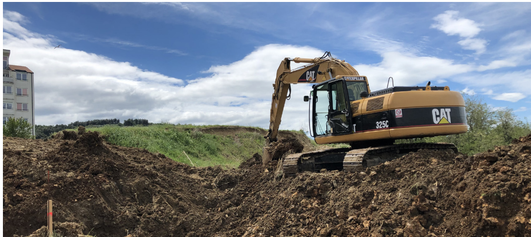
Excavation on the ground in Livade, Izola. Image: Eva Prelovšek Niemelä
